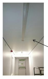
Solid ceiling prevents access to the grease extract which runs directly above the lighting strips. This represents an unknown as further obstructions will be present above the ceiling. Introducing false hatches in obstructed areas may lead to several remedial works being required to correct.
